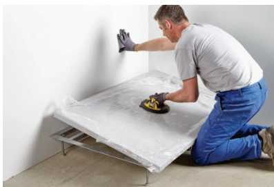
INSTALLATION RECEVEUR
