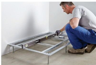
MISE EN PLACE CHASSIS SUPPORT CAREA
